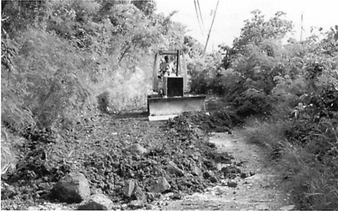
Figure 1: Grading a road segment in St. John, USVI.
