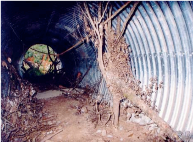
Figure 1. An underpass with natural components to facilitate species movement (Goosem et al., 2005).
